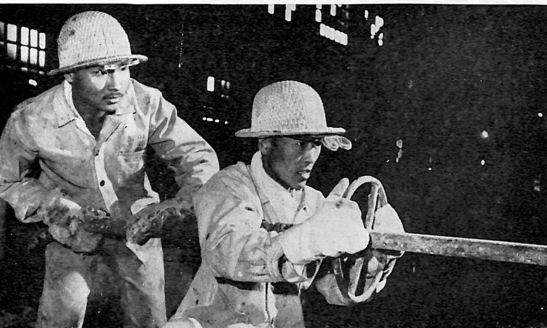
Ignoring the heat, workers repair a converter's brick lining.
